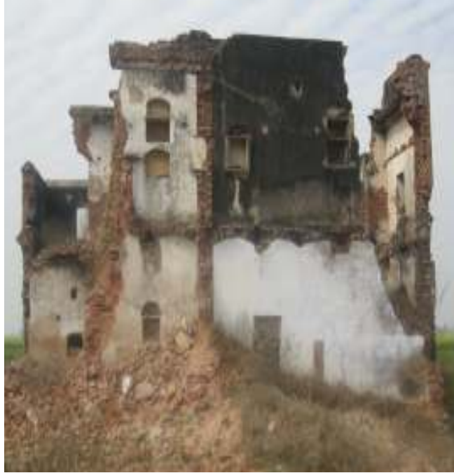
Picture of a burnt house during attack on village Hondh-Chillar, State of Haryana, discovered 26 years after November 1984. Source, File Photo "The Tribune"
